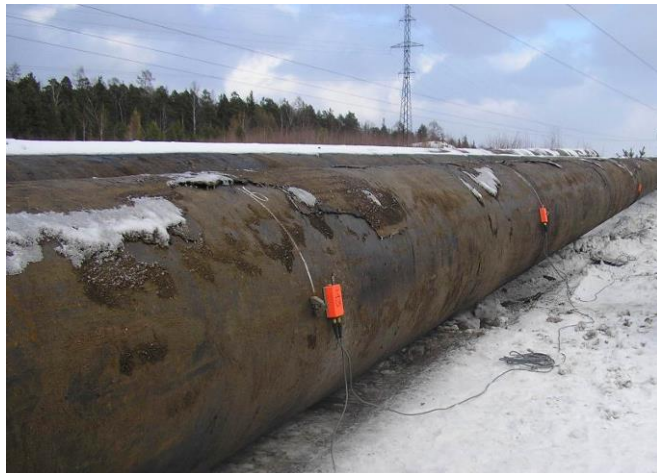
Fig. 3. An experiment on the section of pipeline of length 56 m.
